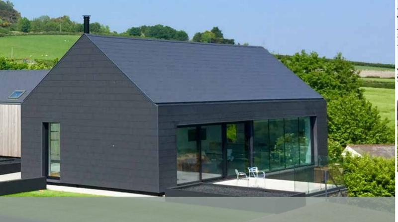
Give free rein to your creativity with vertical slating. A new dimension to design with fibre cement slates.
