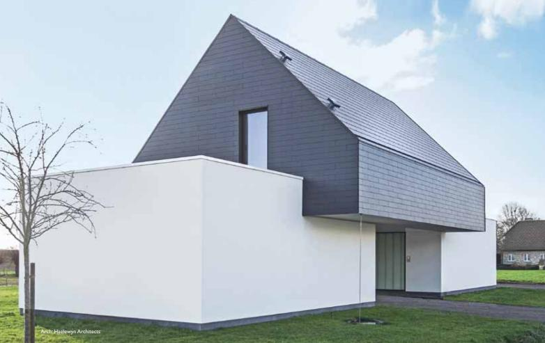
Fibre cement slates can be fixed in varying patterns for unique design.
